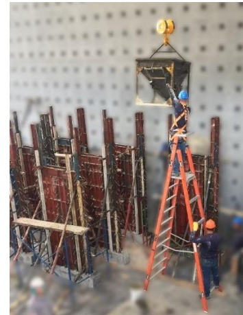
(f) Wall casting
