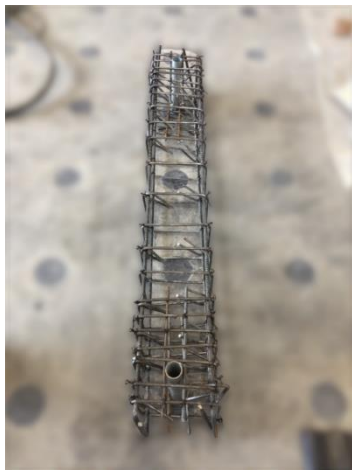
(a) Bottom beam reinforcement
