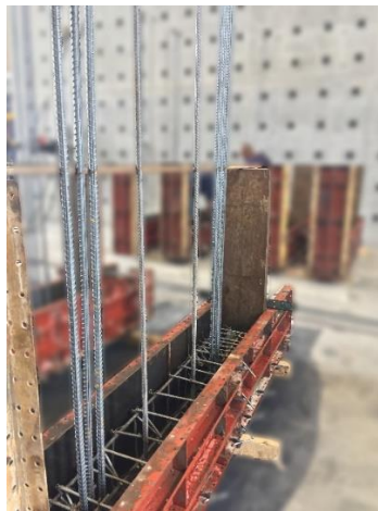
(b) Bottom beam formwork
