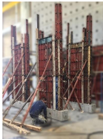
(e) Wall formwork
