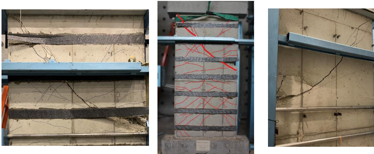
Figure 4.8 – Failure mode H-C1-1 Specimen.
