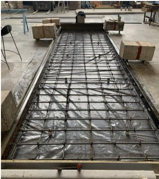
(f) Reinforcing mesh centered on the formwork.
