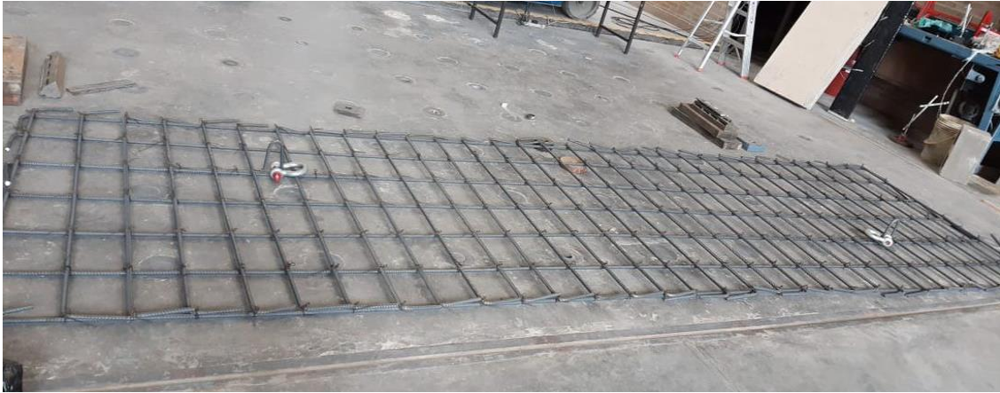
(e) Reinforcing mesh
