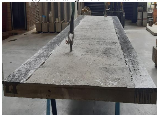
(f) FRP applied.
