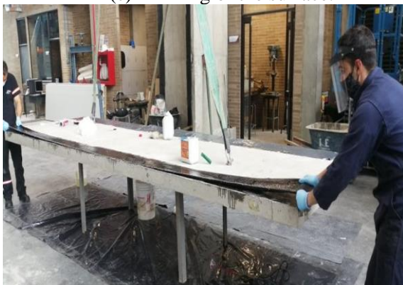
(e) FRP application.
