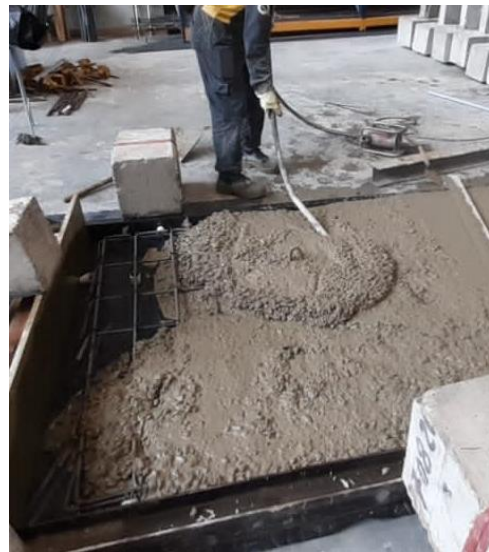
(g) Wall casting
