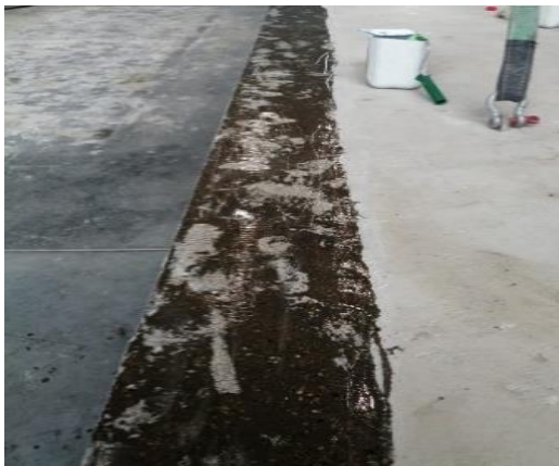
(c) Priming of the surface.
