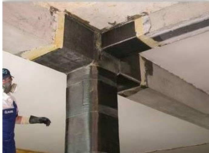
Figure 6. FRP reinforcing beams and columns. Source: Basalto.
