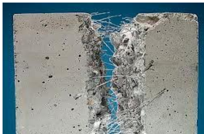
Figure 8. Real image of UHPFRC. Source: IStructe Victoria Branch.
