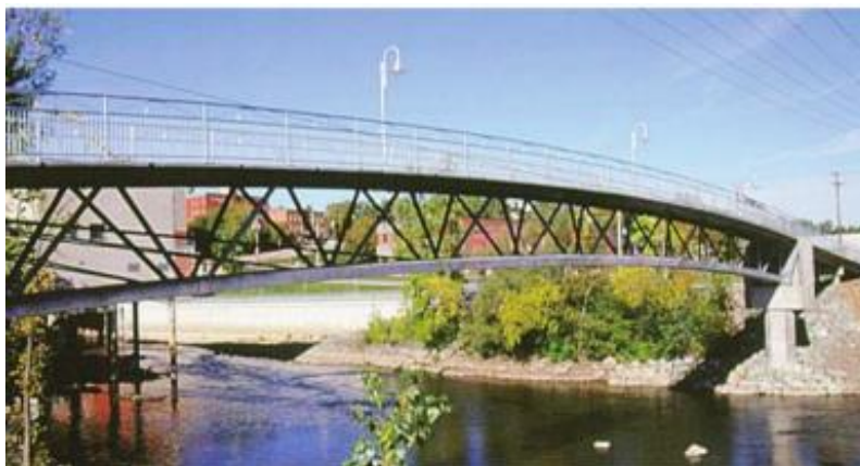
Figura 11 Sherbrooke Pedestrian Bridge (photo courtesy) (ACI, 2018)
