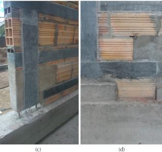
**Figure 3.** Construction process of the anchoring system: (a) removed masonry units and hooked steel bars; (b) placed grout block with bottom gap; (c) installed FRP strip wrapped around grout block; and (d) additional grout filling the gap.
