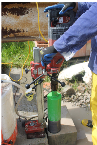
Figure 4. Concrete core extractions.
