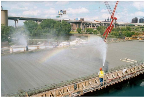
Figure 1. Concrete external curing.
